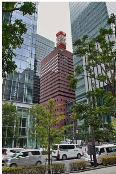
KDDI Otemachi - the first popular interconnection facility
